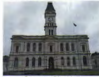
Oamaru City Hall
