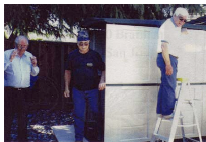
Assembling 2 nd shed & crew
